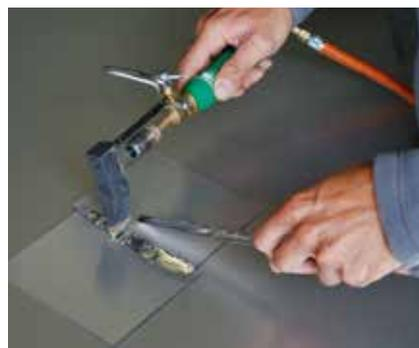
Repeat until soldering joint is completed.
