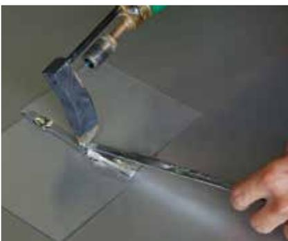
Melt solder, transfer to joint and draw a seam through a continuous movement.
