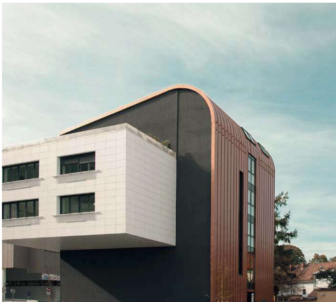
Vile Vodmat - Ljubljana, SLO - 2012 Vestis: rame roof - aggraffatura angolare Vestis: copper roof - angled standing seam
