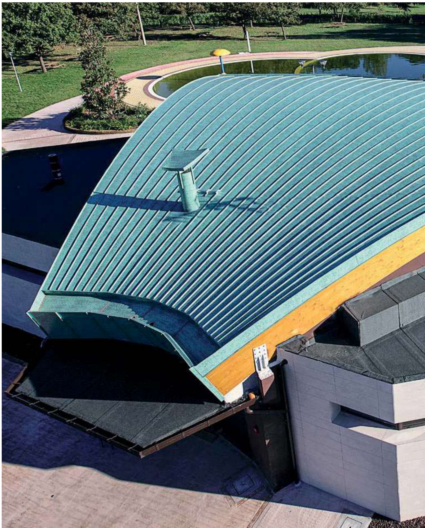
Village Onda Magica - Castropignano, IT - 2013 Vestis: verde roof - doppia aggraffatura Vestis: green roof - double standing seam
